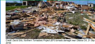
Credit: David Sills, Northern Tornadoes Project (EF3 tornado damage near Ottawa CA, 21 Sep 2018)
